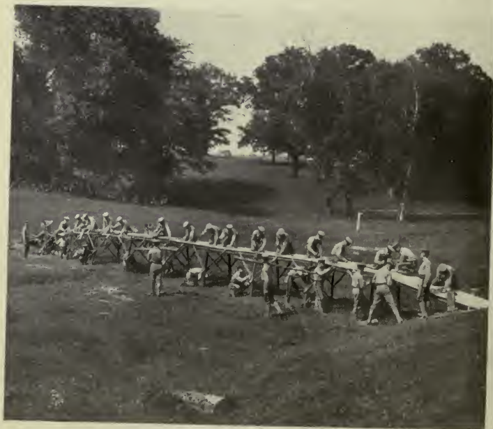
Instruction in Trestle Bridge Building—Western
